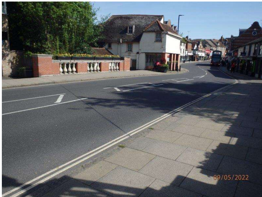
2 – View of east approach to bridge
