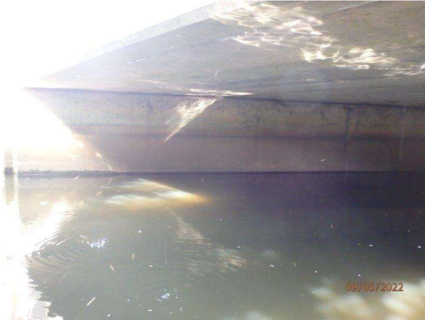
7- Soffit of the deck
