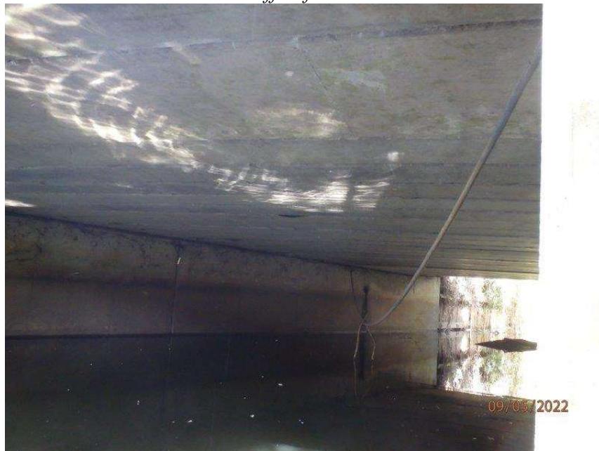
8- Soffit of the deck
