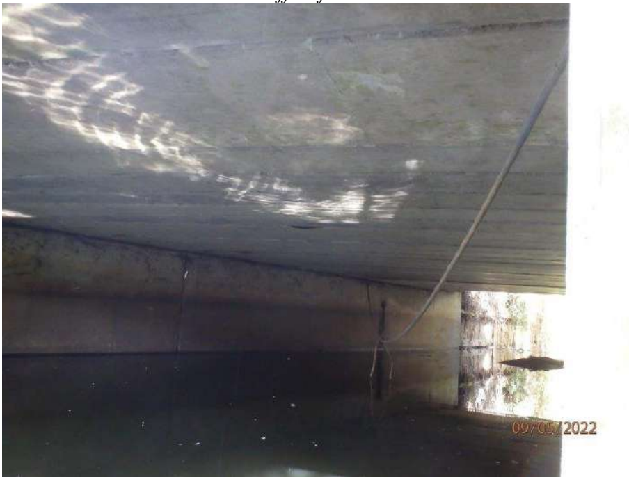
8- Soffit of the deck
