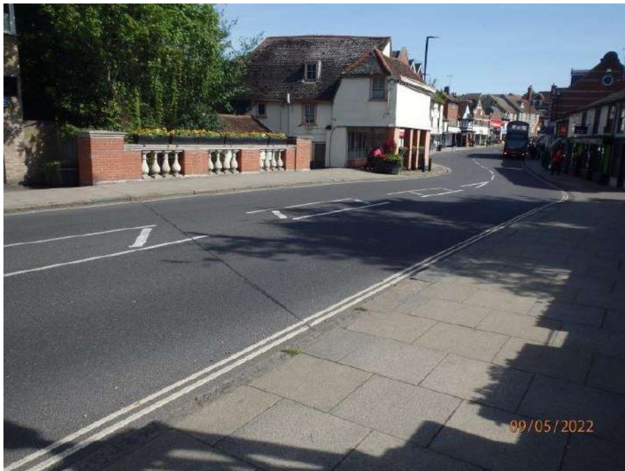
2 – View of east approach to bridge
