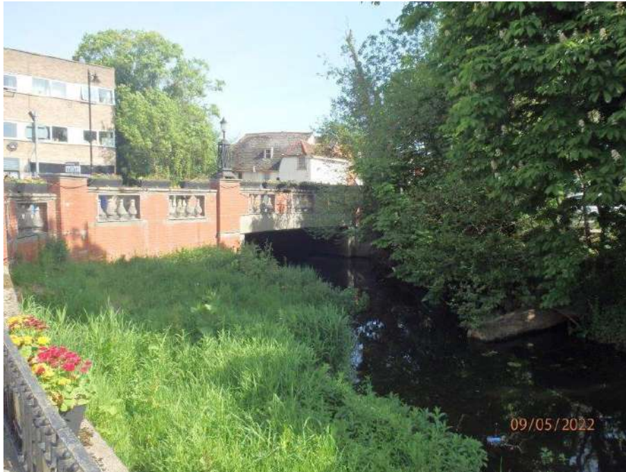
1 – View of bridge from south
