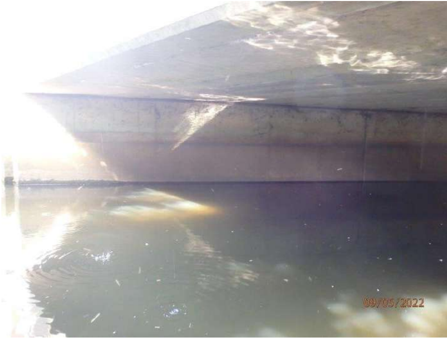
7- Soffit of the deck
