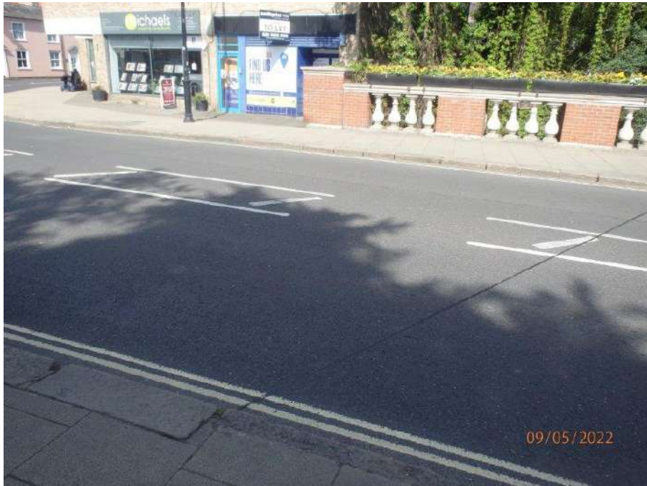
4 – Top surface of bridge
