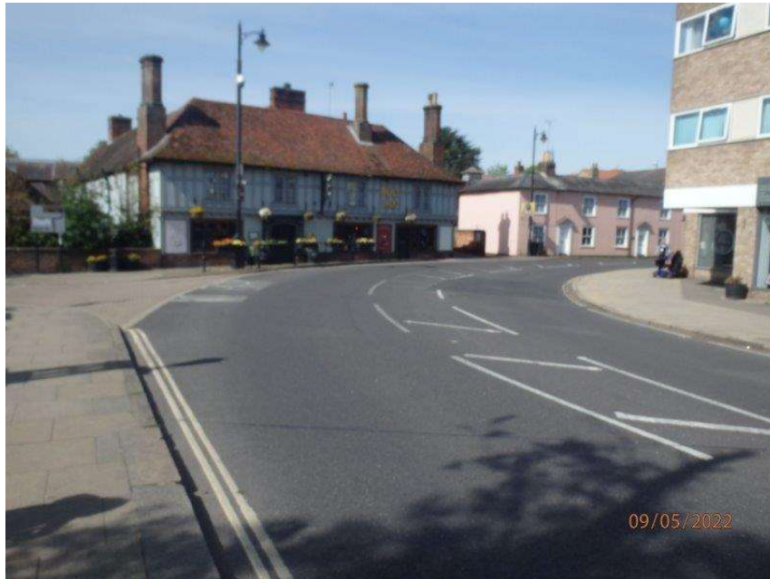
3 – View of west approach to bridge
