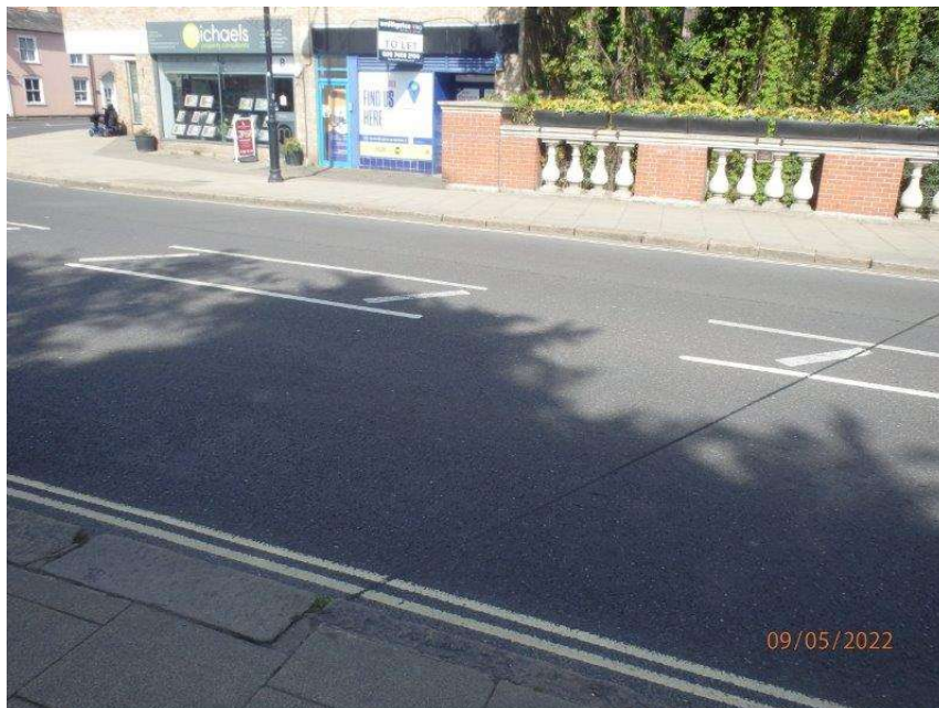
4 – Top surface of bridge
