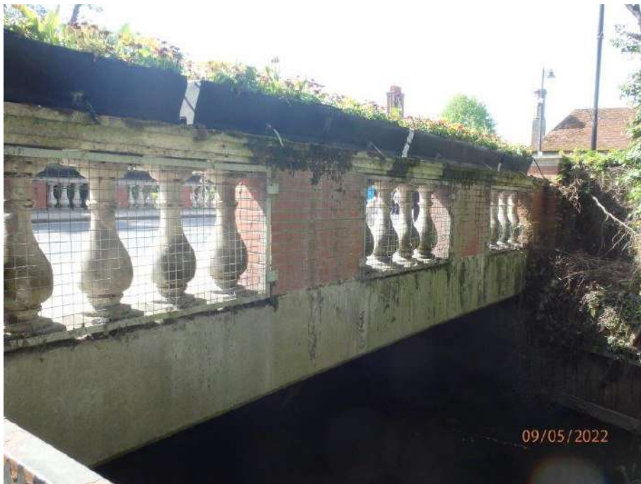
6 – North side of bridge
