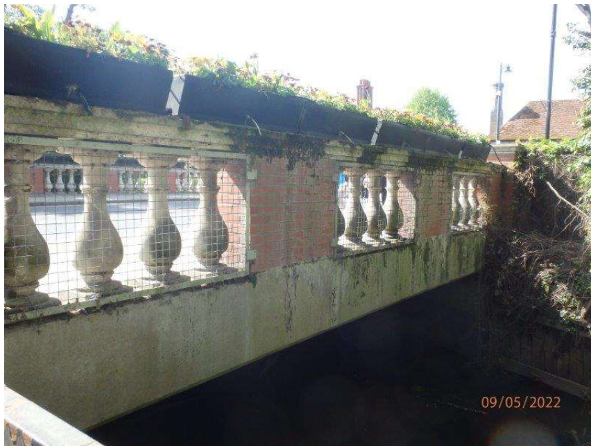
6 – North side of bridge
