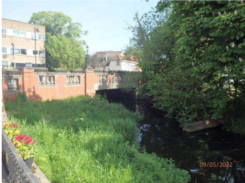
1 – View of bridge from south
