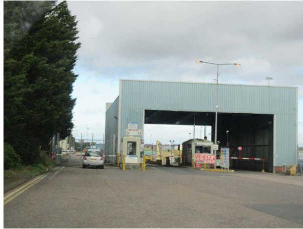
Photograph 36 Port Exit at West Bank. Gate width 5.4m. Negotiable.
